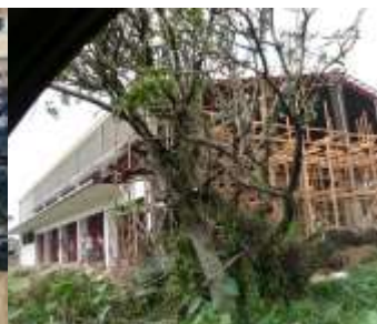
New building nearing completion, March 2010
